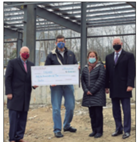
The campaign for the construction of the Adaptive Wellness Center by Favarh, the Arc in the Farmington Valley, recently received a $35,000 donation from Collinsville Bank , a division of Northwest Community Bank. The Center is being created to provide the individuals Favarh serves more opportunities to enjoy a healthy and active lifestyle. The Center will include a large multi-use floor to be used for a variety of mindfulness activities, sports, recreation and theater programs.
